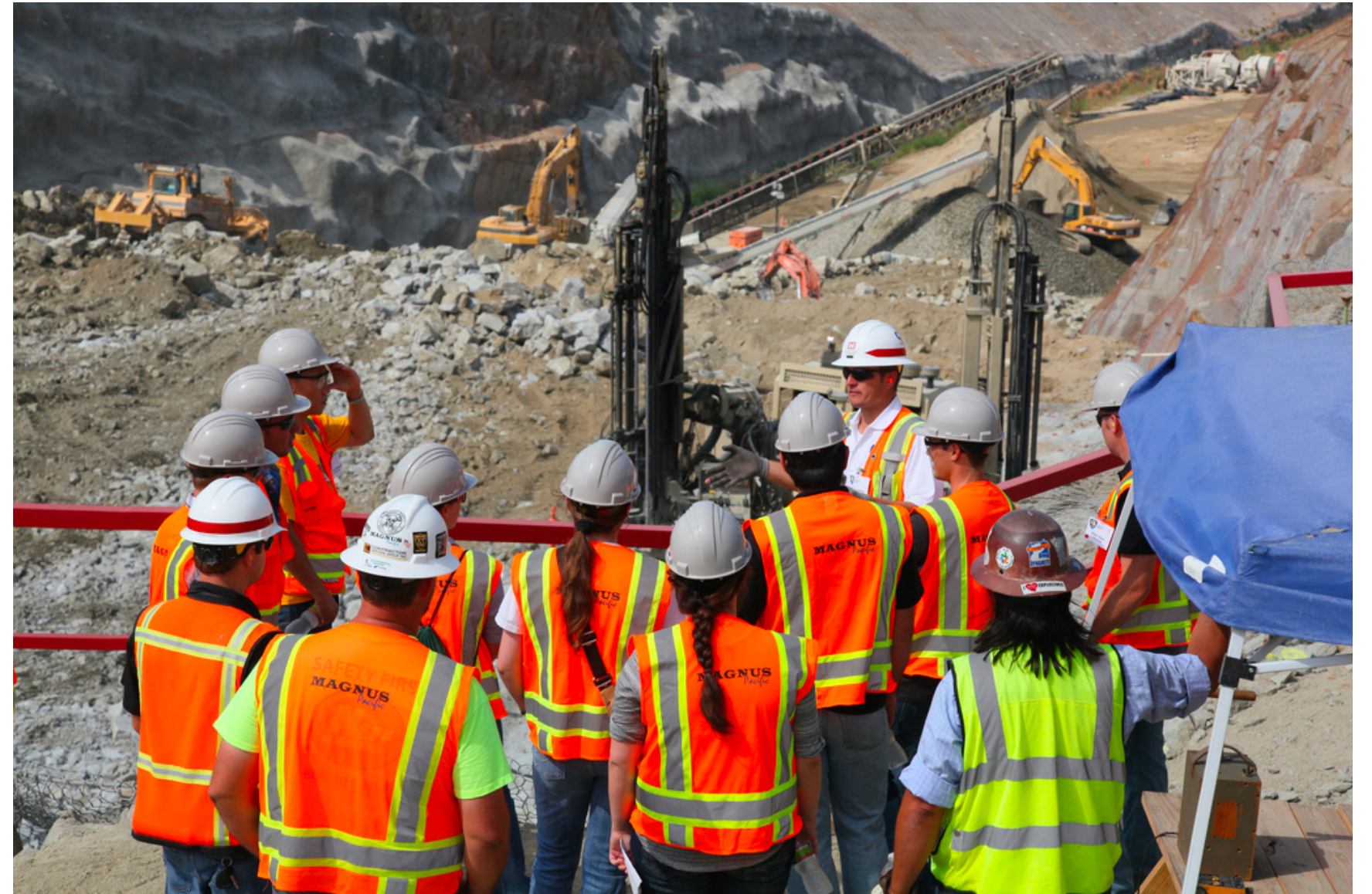
"Construction and engineering students visit the Folsom spillway job site" by USACE HQ is marked with Public Domain Mark 1.0.
